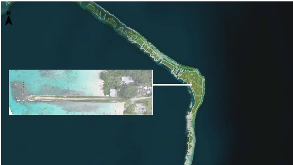
Figure 1-5: Wotje works location
