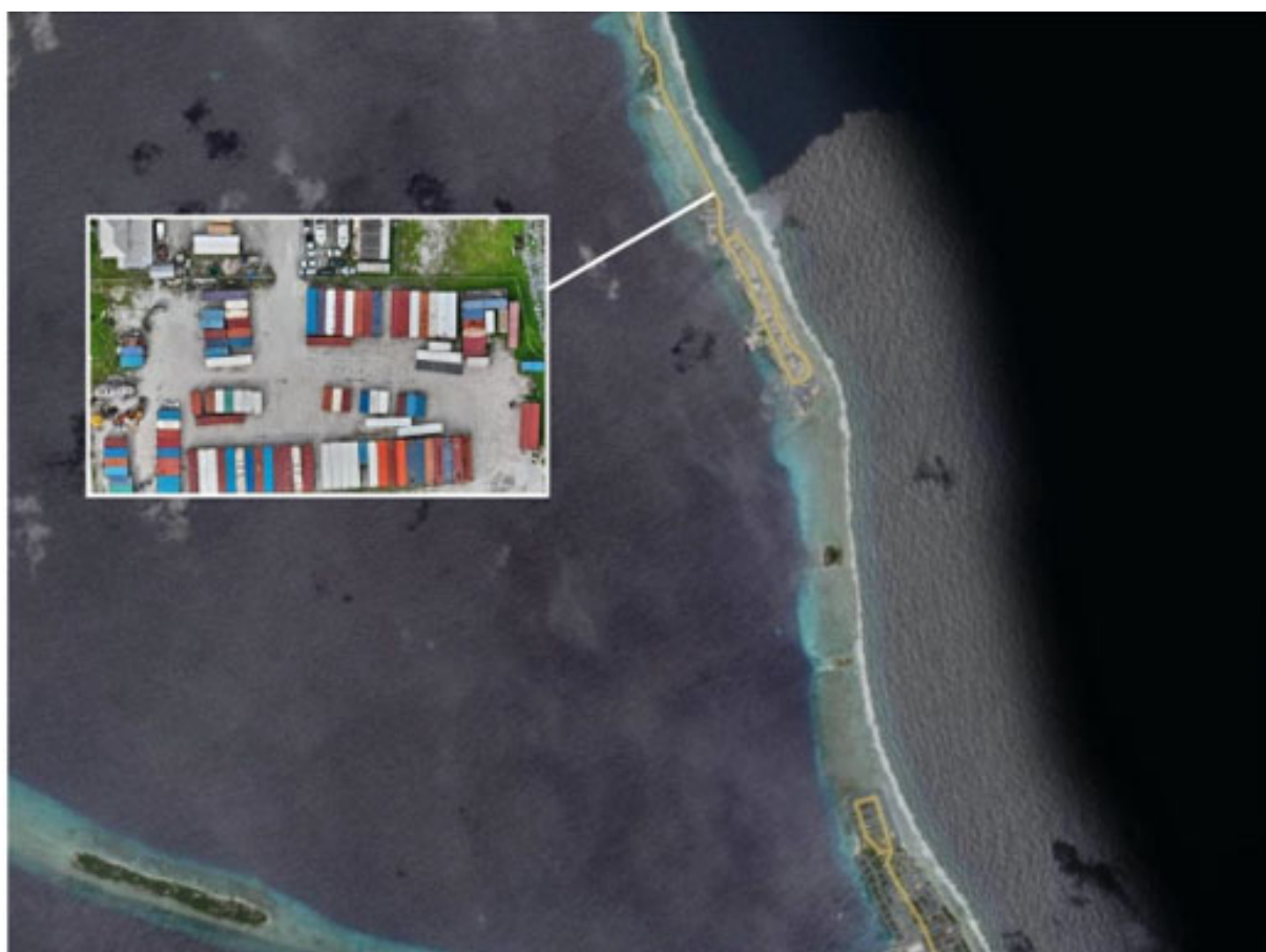
Figure 1-2: Ebeye works location
