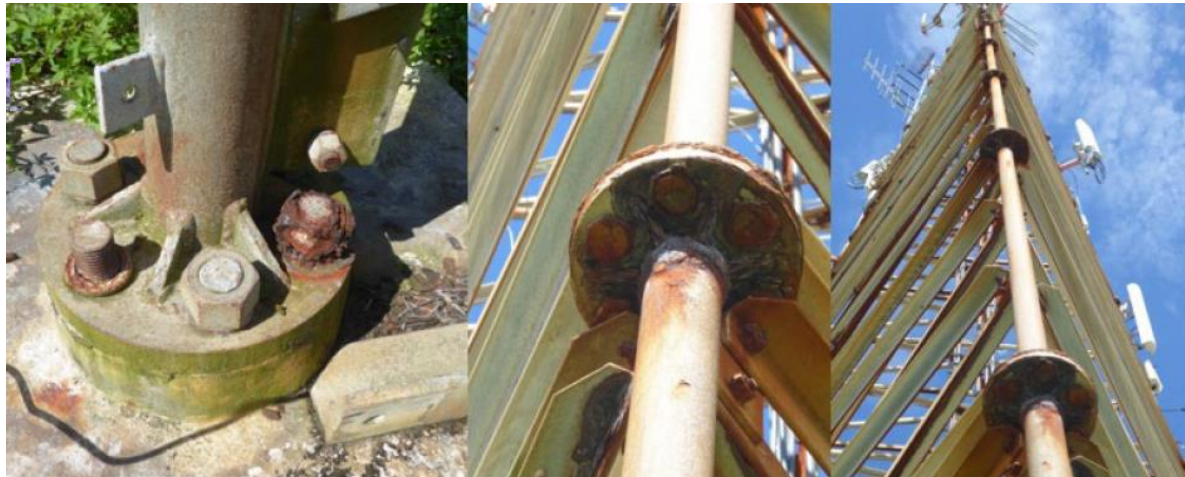
Figure 13 - Condition of Majuro Towers 2017/8
