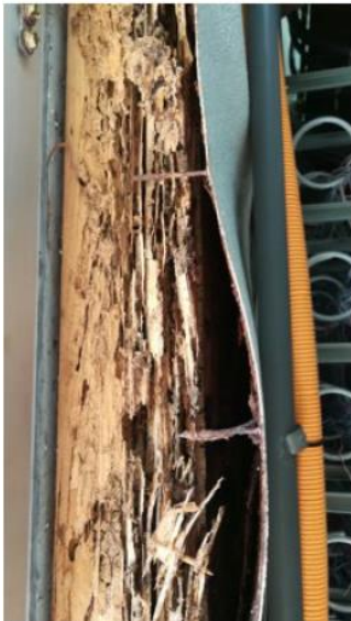
Damaged-internal-insulation
