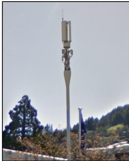
Figure 7: Example of upgraded mobile tower in Queenstown NZ. Multiple frequencies have been added to provide Gigabit throughput.
